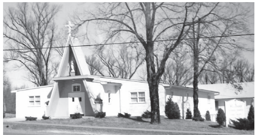
The original St. Ann Church in Warsaw was renovated and built onto several times before the current church was built in 1995.
